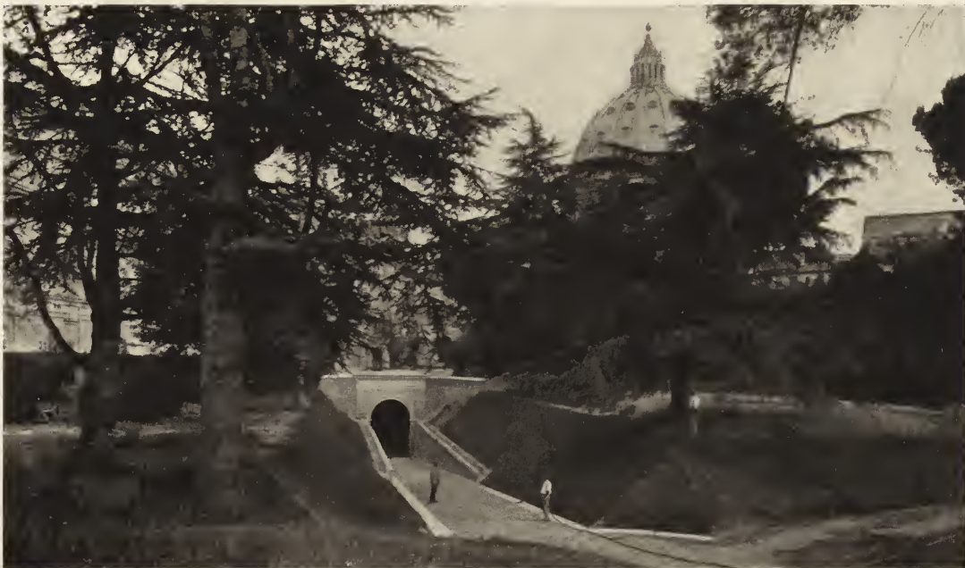
Exit of Tunnel
